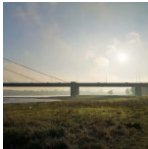
Blick zur Theodor-Heuss-Brücke
